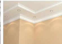
Siling Plaster Plaster Ceiling 石膏天花板
