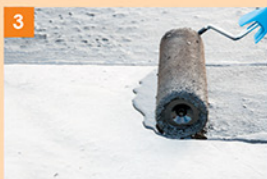
3 Apply with brush, roller or spray 用滚筒, 喷涂或刷子均匀涂布
