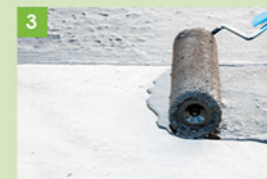
3 Apply with brush, roller or spray 用滚筒, 喷涂或刷子均匀涂布
