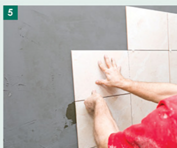
5 Finish with tile 涂布完成后并铺盖瓷砖
